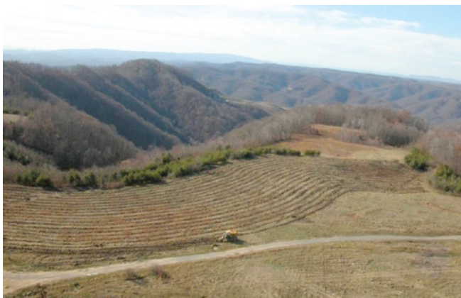
Figure 10. An aerial view of a former mine site being prepared for reforestation. Woody vegetation was removed and herbaceous vegetation was herbicided prior to the deep-tillage operation shown by the photo. Photo by Richard Davis, Virginia Department of Mines, Minerals and Energy.
